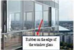
Figure 2.3. Installing Rubber on the Edges of Window Glass
