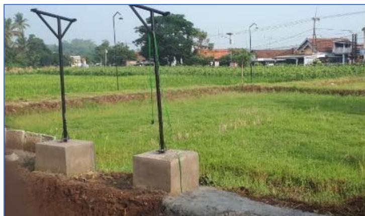
Gambar 23 Pemasangan Tiang Panel Surya
