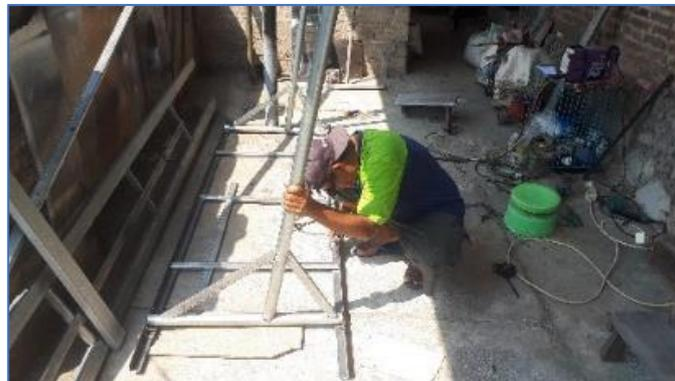
Gambar 19 Pengelasan Tiang panel Surya
