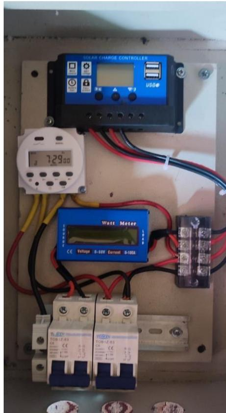
Gambar 6. Instalasi Sistem Kontrol Panel Surya
