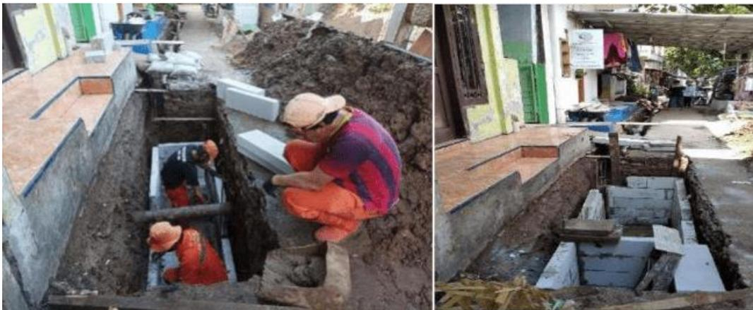
Gambar 4. Pemasangan dinding Septik tank
